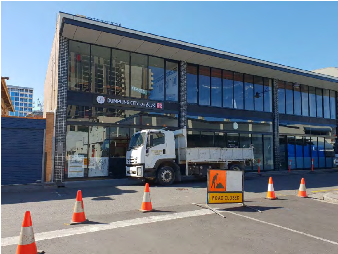
Photo 3 – New development on east side of Field Street
